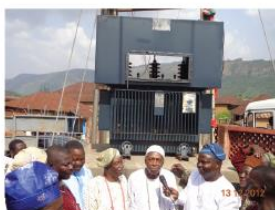
Moro 7.5MVA, 3311KV Power Transformer
