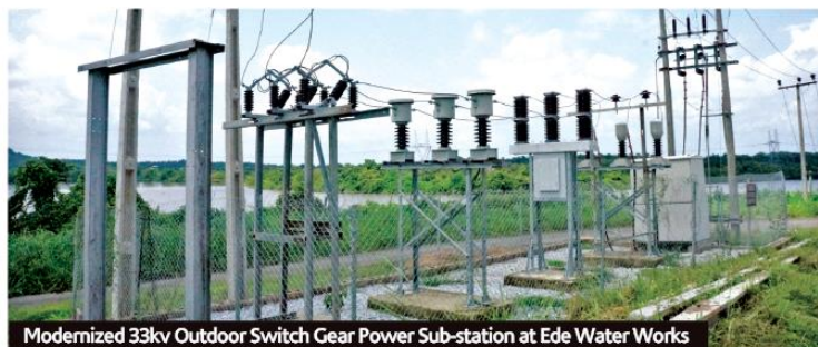
Modernized 33kv Outdoor Switch Gear Power Sub-station at Ede Water Works
