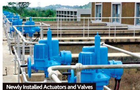
Newly Installed Actuators and Valves
