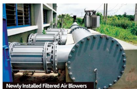
Newly Installed Filtered Air Blowers
